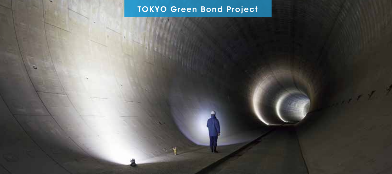
Kandagawa River Ring Road No.7 Underground Regulating Reservoir (underground tunnel type)
