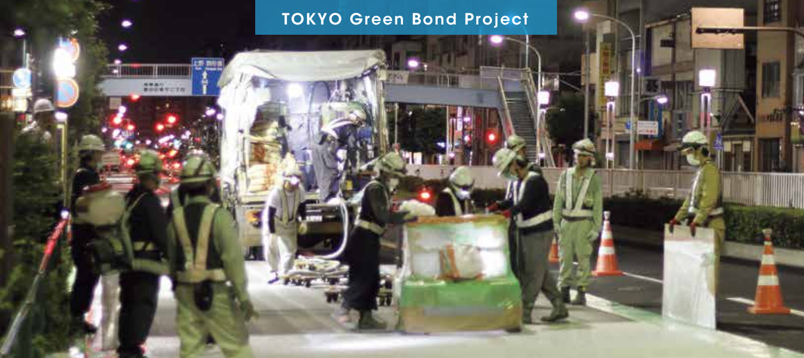
Heat-insulation paving works on road surface
